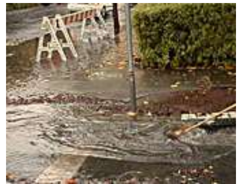
Photos of stormwater drains with leaves blocking flow and stormwater drain after rainfall backing up into roadway
