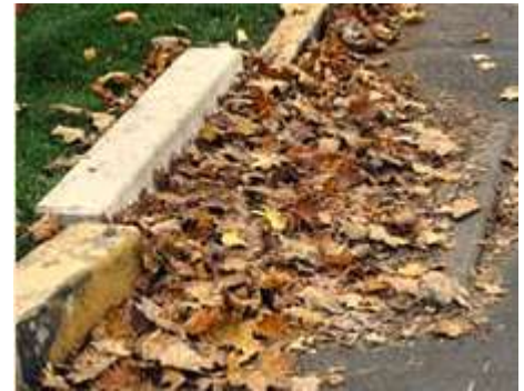
Photos of stormwater drains with leaves blocking flow and stormwater drain after rainfall backing up into roadway
